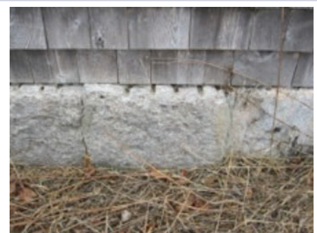
Stone splitting marks visible from plug drill – post 1830.
