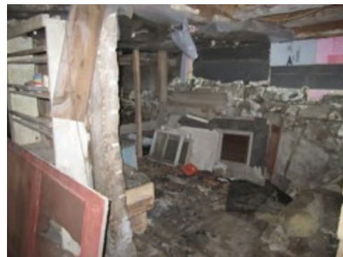
Basement: a variety of insulation can be seen on the foundation wall and the granite post with its splitting marks.
