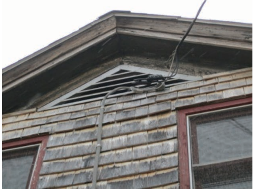
Trim detail covered by wood shingles.
